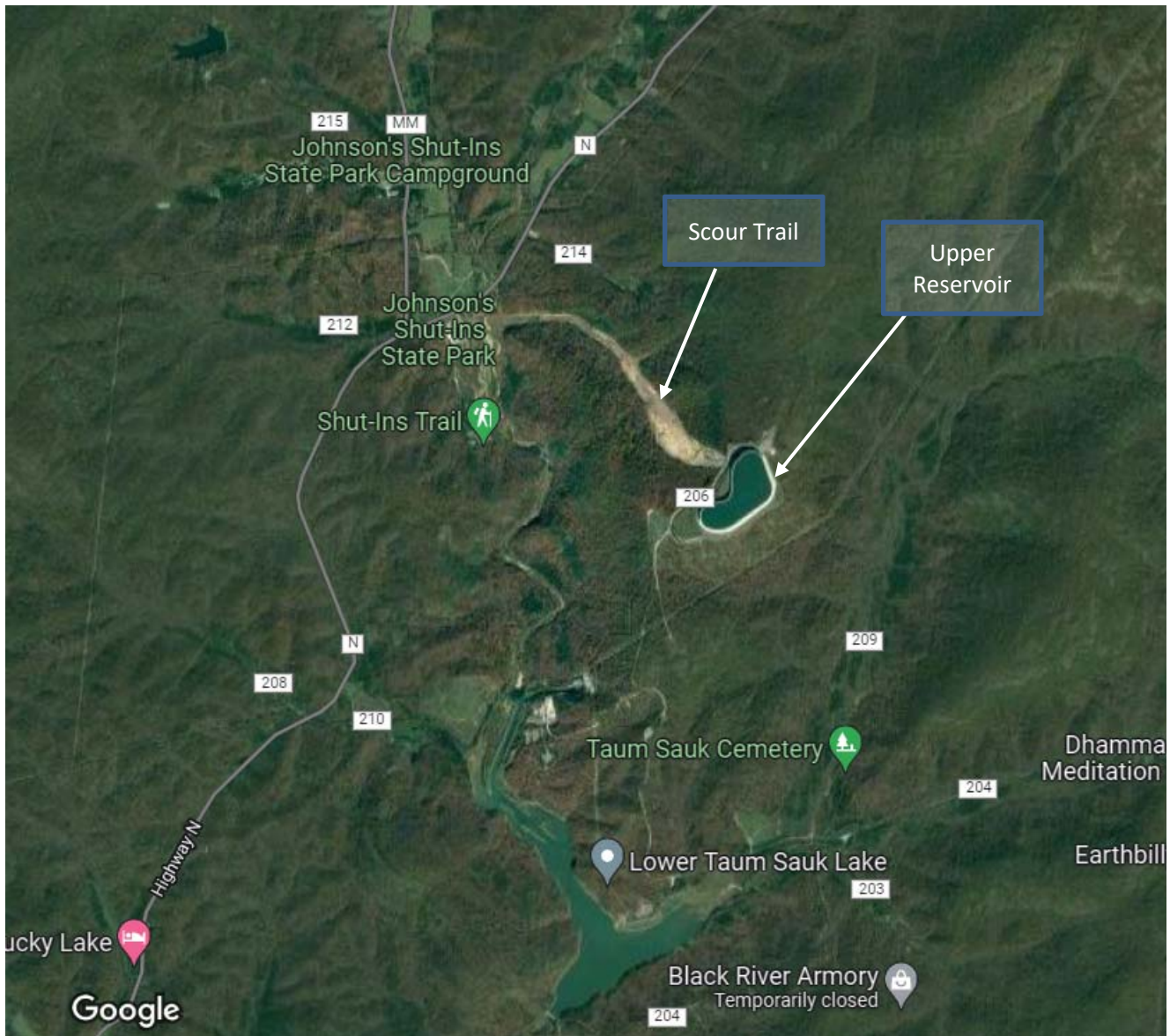
Figure 3.6. Aerial View of Taum Sauk Upper Reservoir Breach, Reynolds County, Missouri
