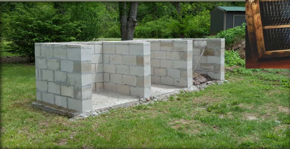
Doniphan Community Composting Station
